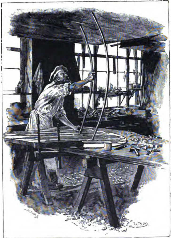
STRENGTHENING A SOUNDING-BOARD: USING GOBARS.
